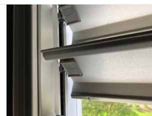
Figure 3. Close view of the exterior blinds with halved hexagonal shape.
